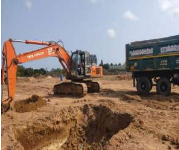
Earth work Excavation
