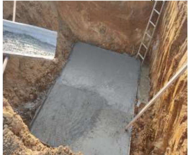
PCC Concrete Work
