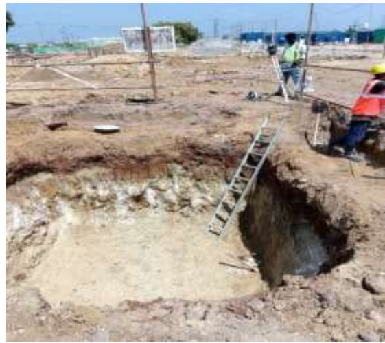
Footing Levelling and PCC Marking Work
