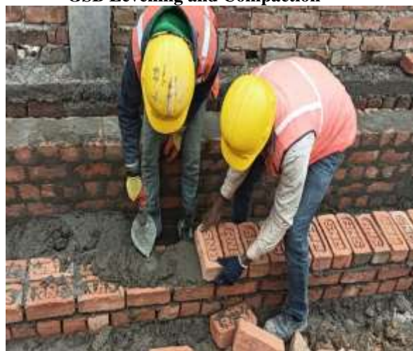
Brick/ Block Work
