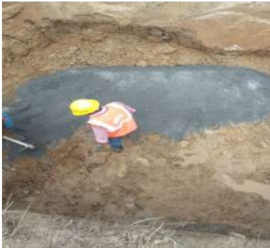
M- Sand Filling Work
