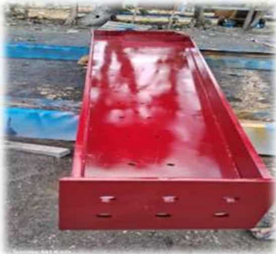
MS Structure Painting
