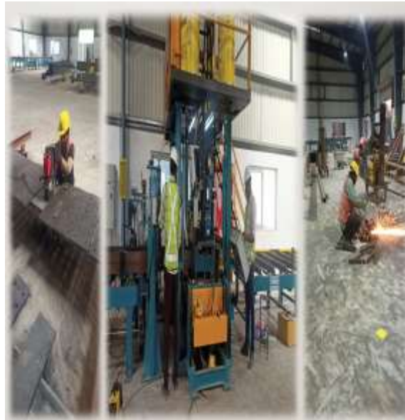
Civil Foundation Fabrication Work
