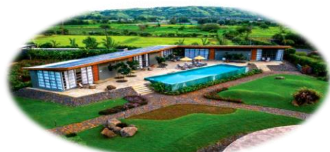
The “Beyond by Sula” facility in Nashik
