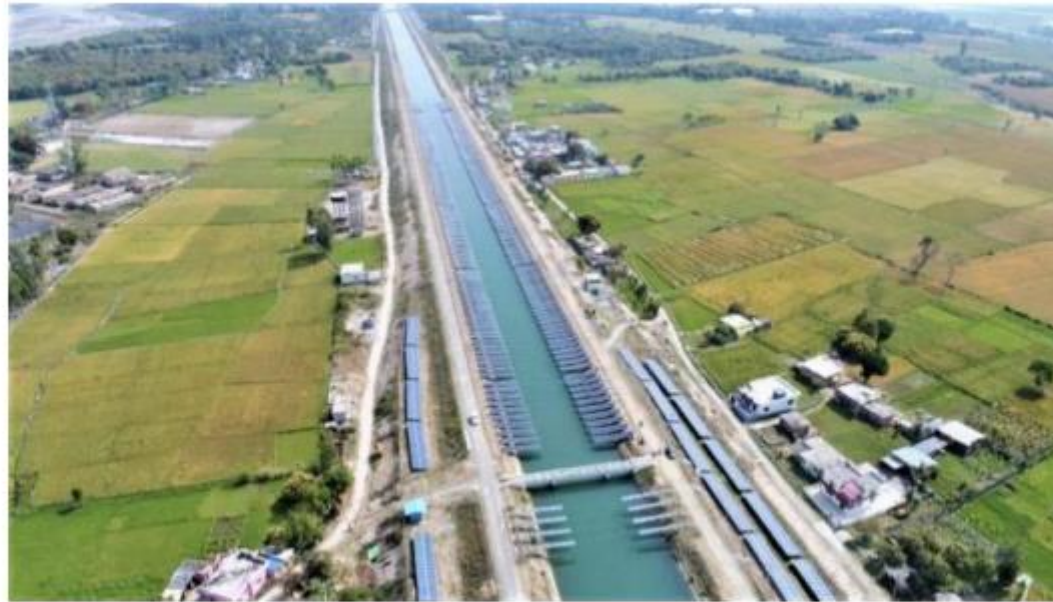
Canal top solar power plant on 35-meter-wide Yamuna Power Channel in Uttarakhand installed by our Company using suspension rope technology
