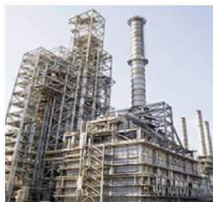
Catalytic Reforming Heaters
